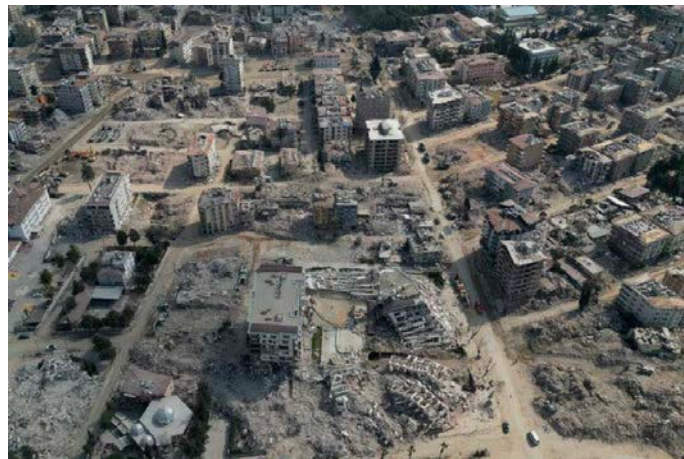
The collapsed Guclu Bahce complex in Antakya, Turkey, in March. Sergey Ponomarev for The New York Times
