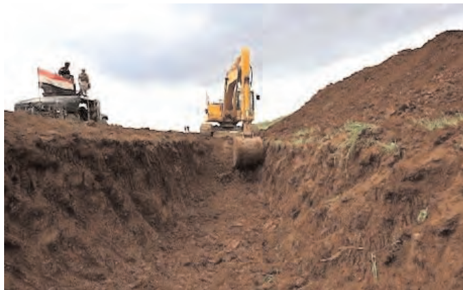
Officials say the trench is three meters wide and two meters deep, aimed at preventing smugglers and terrorists from infiltrating into Kurdistan. Photo: Rudaw
