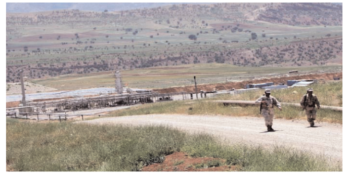
Two armed security guards check oil pipeline in an oil field in Kurdistan region of northern Iraq.
