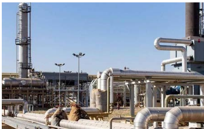
Khor Mor gas field in Sulaimani province's Chamchamal district. Photo: File/Dana Gas
